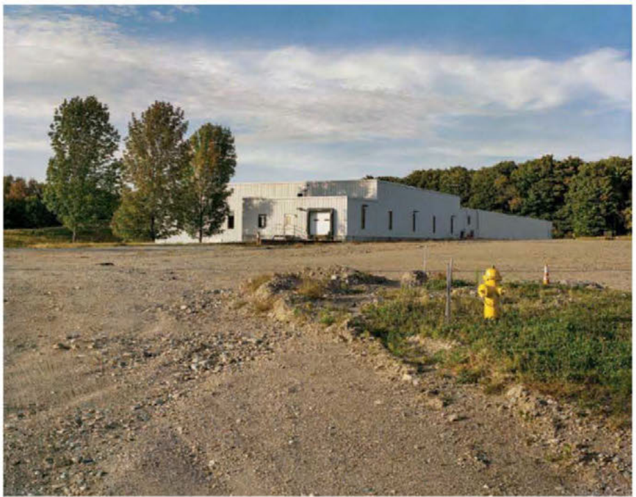
The abandoned site where Stenger and Quiros promised to create a biotech center
